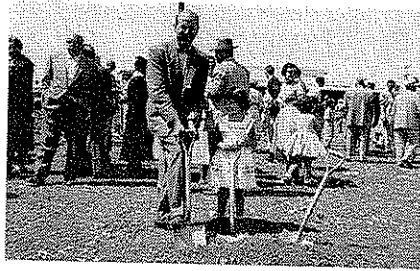
Charlie Mandel and daughter Mimi at the 1955 groundbreaking for the present Temple site.
